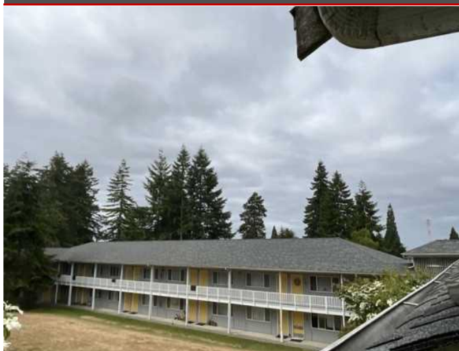
7 - PRIMARY ROOF OVERVIEW
