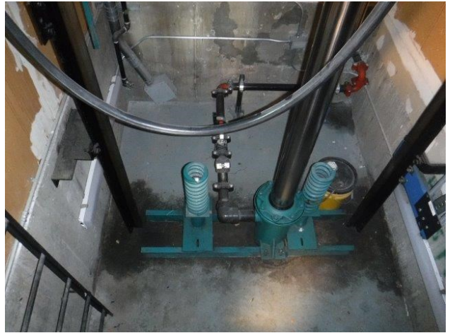
2. Pits are clean.
