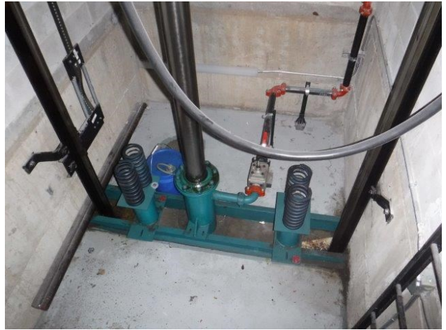
2. Pits are clean.
