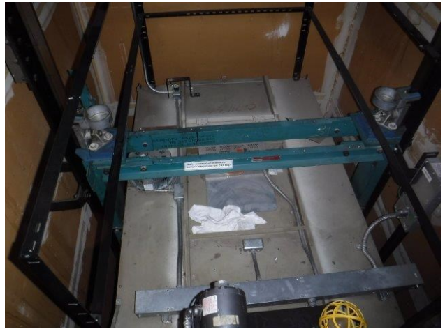
4. Fill lubricator reservoirs.
