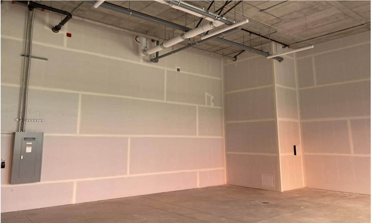
Above: looking southwest from inside Space C.
