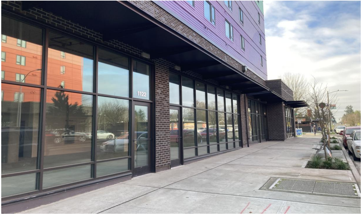
Above: looking southwest at front windows and doors from 11 th St.
