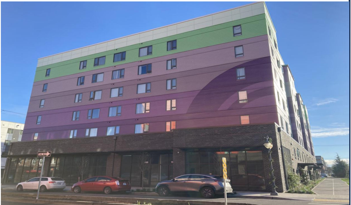
Above: looking south at overall building front windows and doors.
