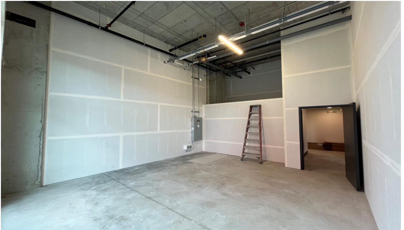
Above: looking southeast to space and bathroom access of Space B.
