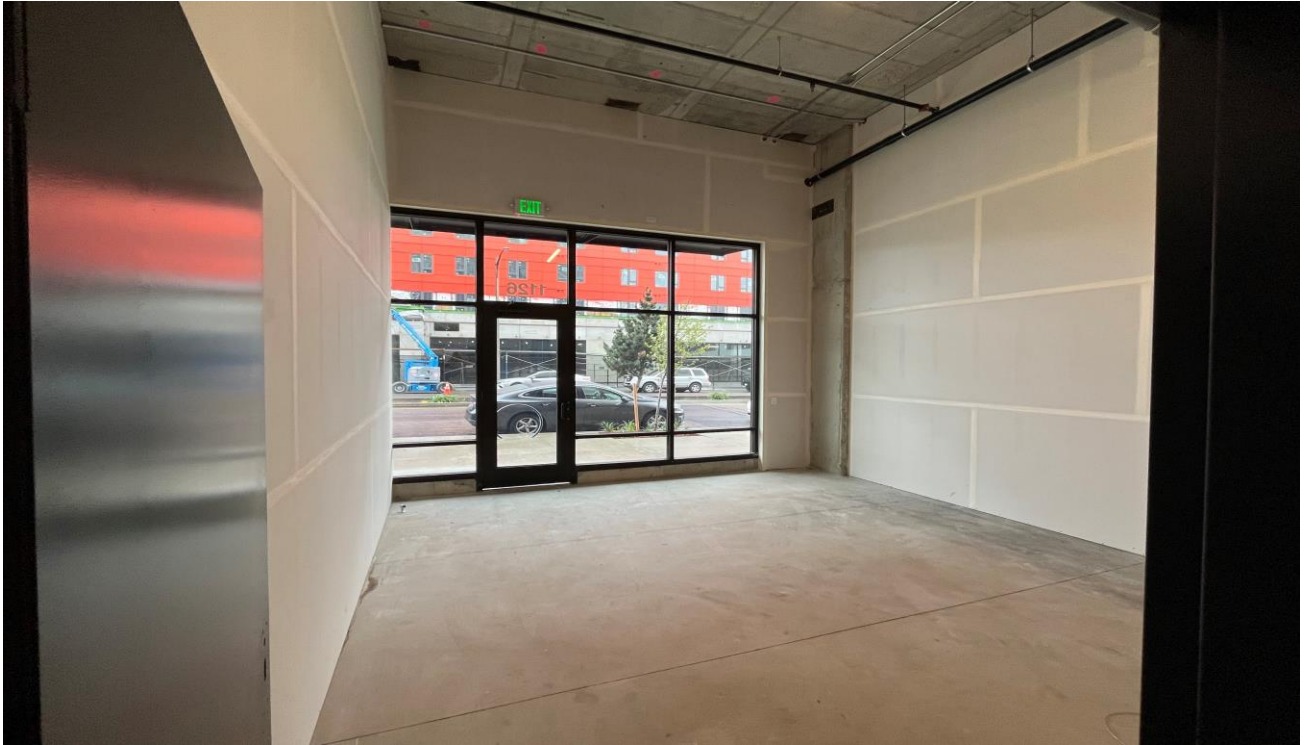
Above: looking north in Space B to entrance.
