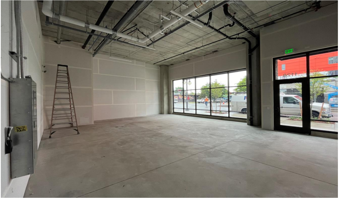
Above: looking northwest at Space C.
