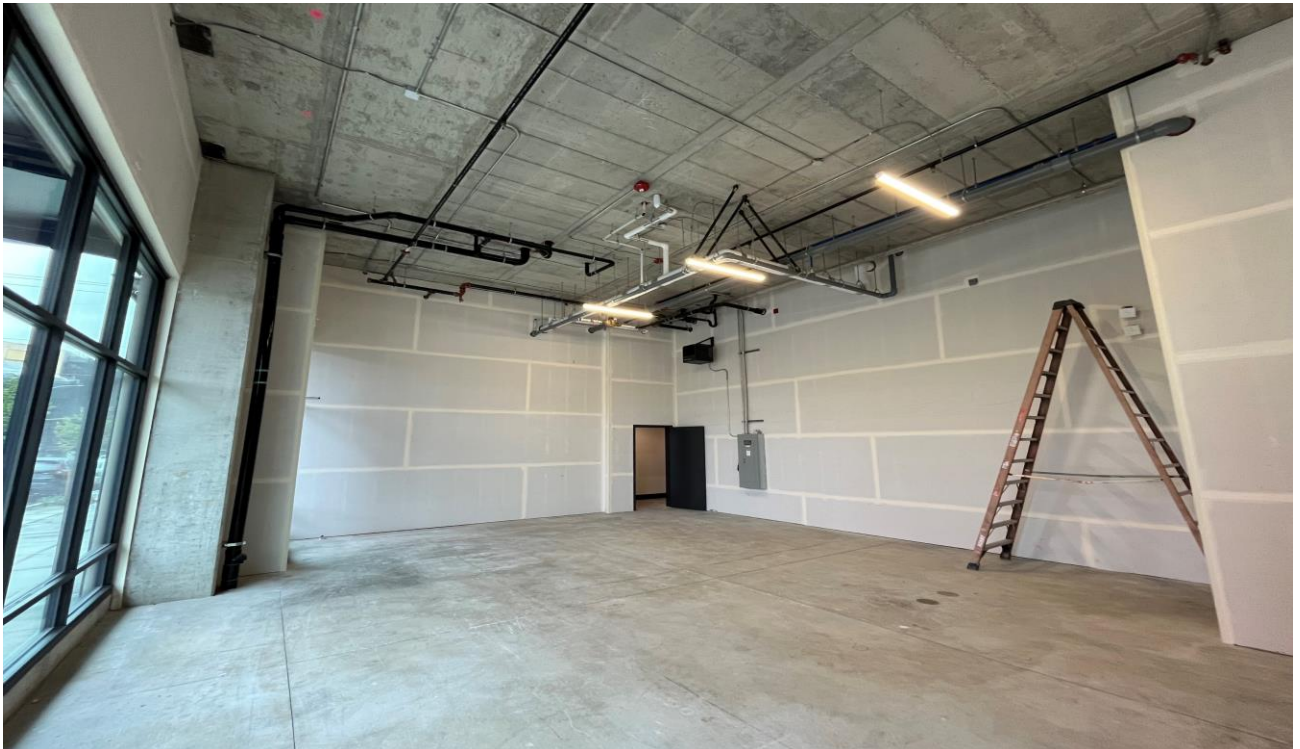
Above: looking southeast to bathroom/hallway from inside Space C.
