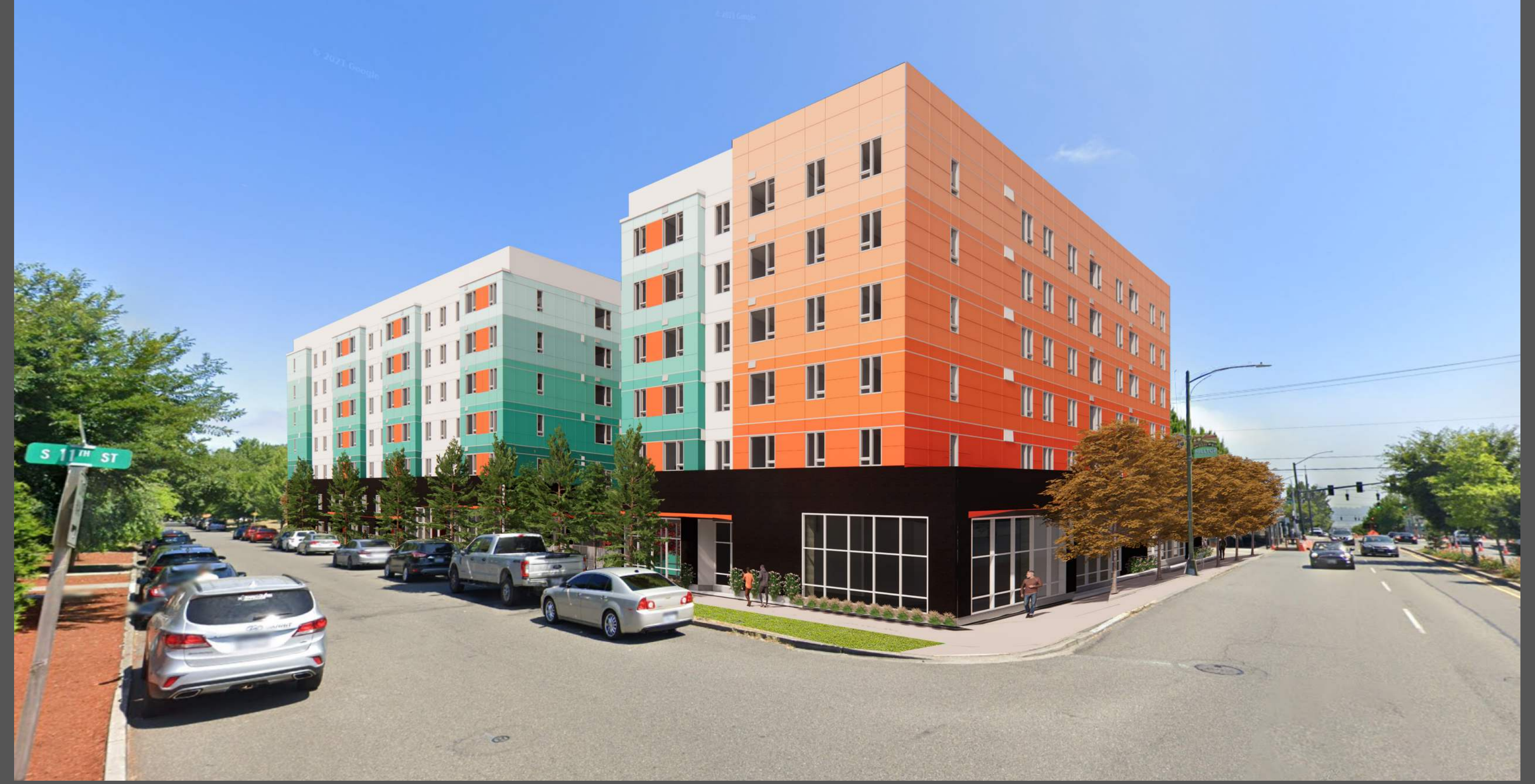
VIEW D: FROM S L STREET & S 11TH STREET LOOKING NORTHEAST
