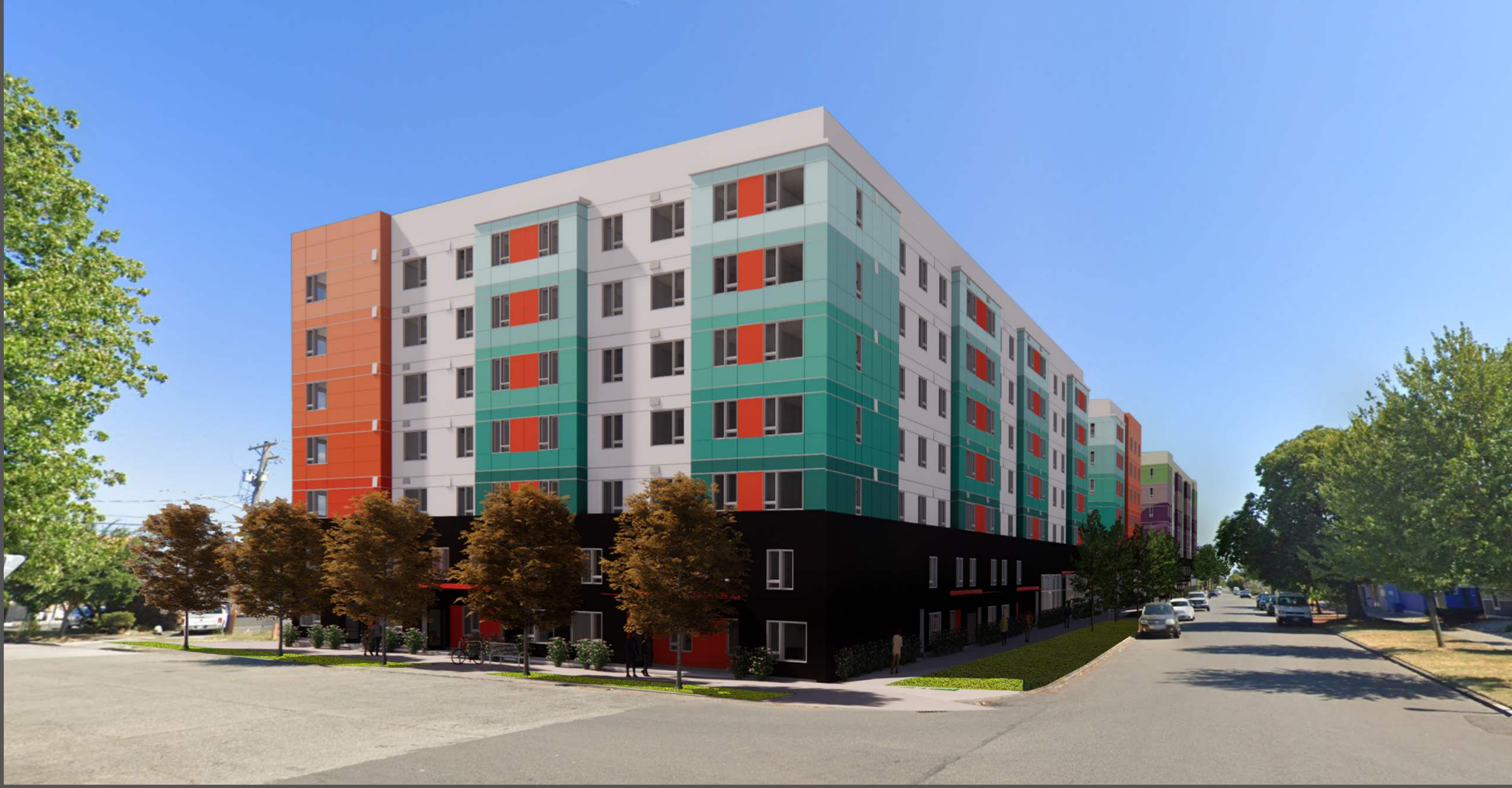
VIEW C: FROM S L STREET & S 10TH STREET LOOKING SOUTHEAST
